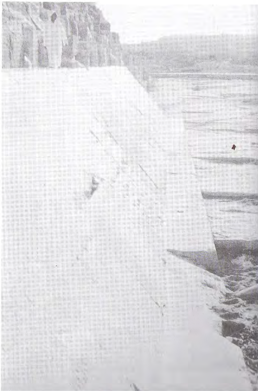
Close up of Great Pyramid showing remaining casing blocks at its base. Courtesy of Wayne Chandler and Gaynell Catherine.
