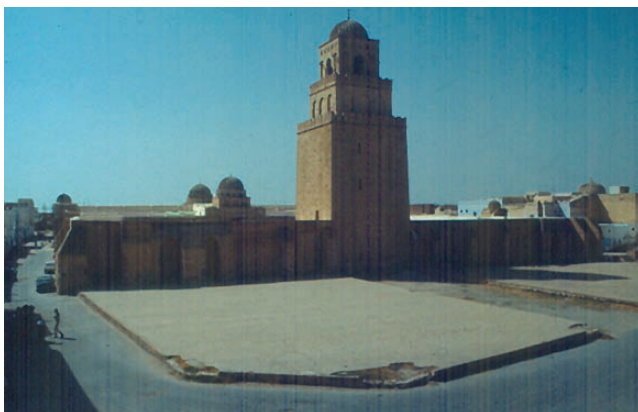
Fig. 7 The Great Mosque of Qayrawan
